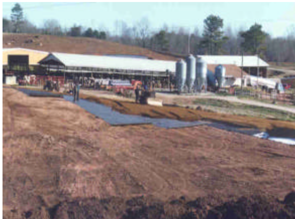
Heavy Use Area Under Construction Ray Haynes & Sons Farm
