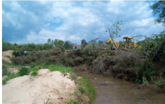
After a mixture of large and small trees have been placed on the eroded streambank, the trees are tightly compacted into a dense mat on the eroding streambank.
