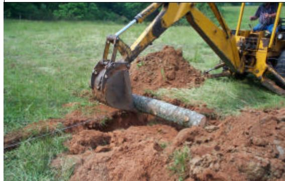
The tree revetment is then anchored in place using cables attached to a log called a "deadman" which is then stretched tight and buried approximately 15' away from the streambank.
